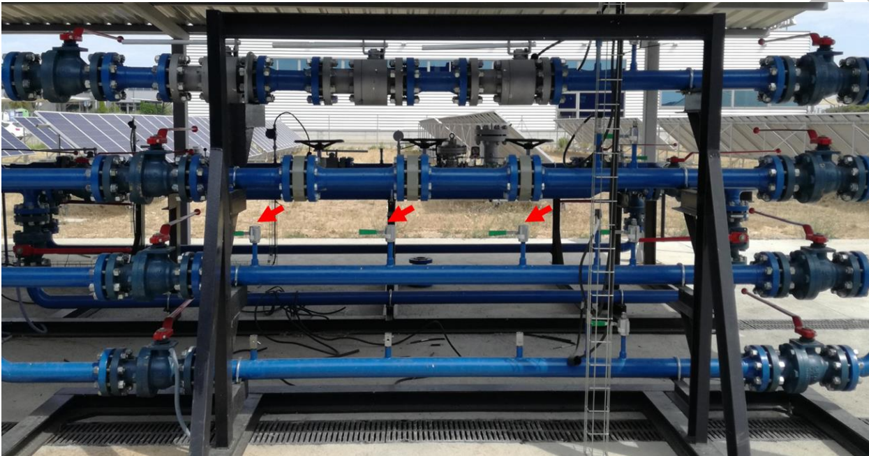
Figure 25. Picture of part of the static section of the testing platform. Red arrows show the point where hydrogen leakages were detected
